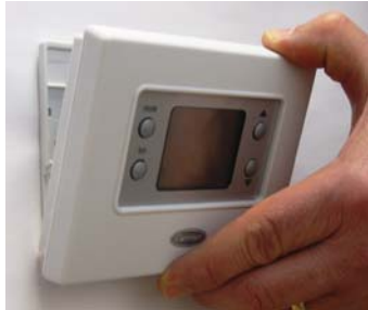
Fig. 4 - Attach Comfort Series Programmable Thermostat
